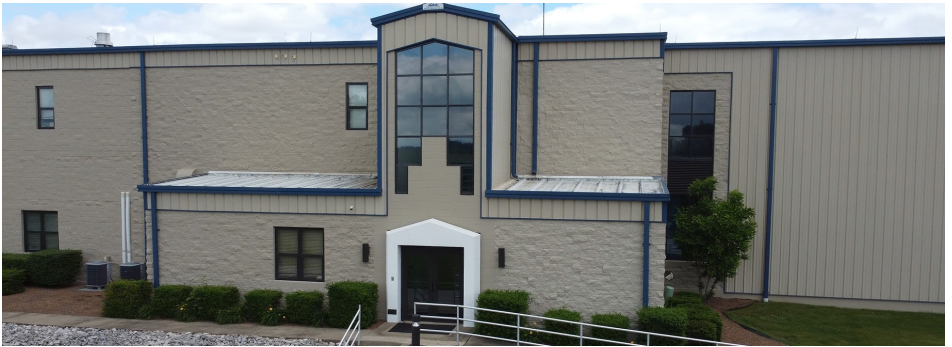
White Mills Water Treatment Plant
